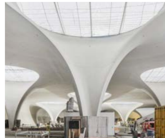
Referentie treinstation Stuttgart - daglichttoetreding
